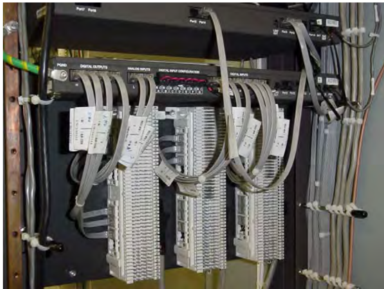
FIGURE 9-19 EXAMPLE OF CABLE LABELING
